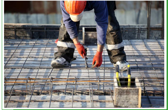
armature metalliche passo 20cm by Rossi ing. Antonio (DL)
